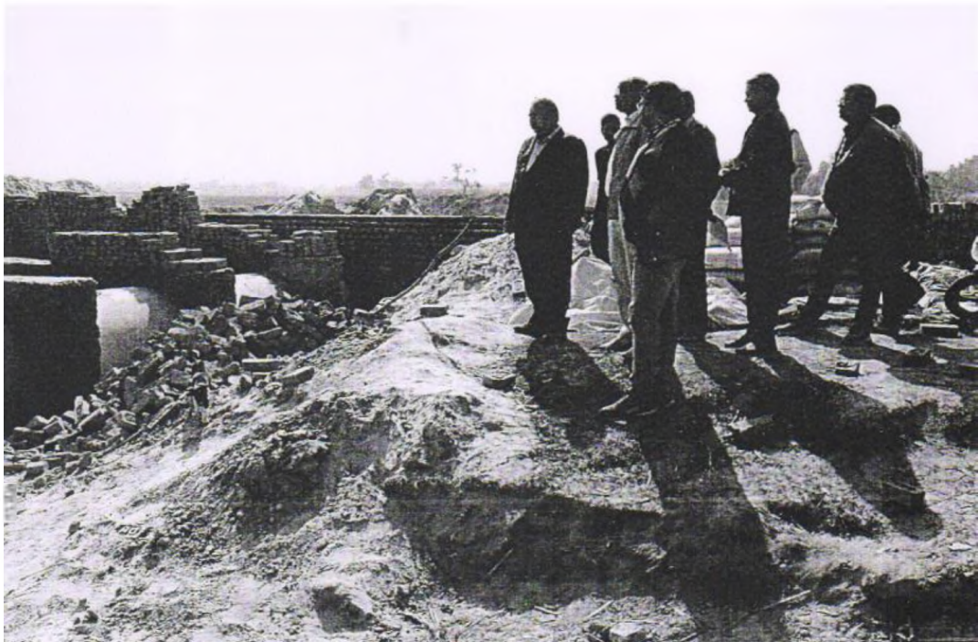
Elgin Bridge Embankment(UP-27)- Barabanki(U.P.)
