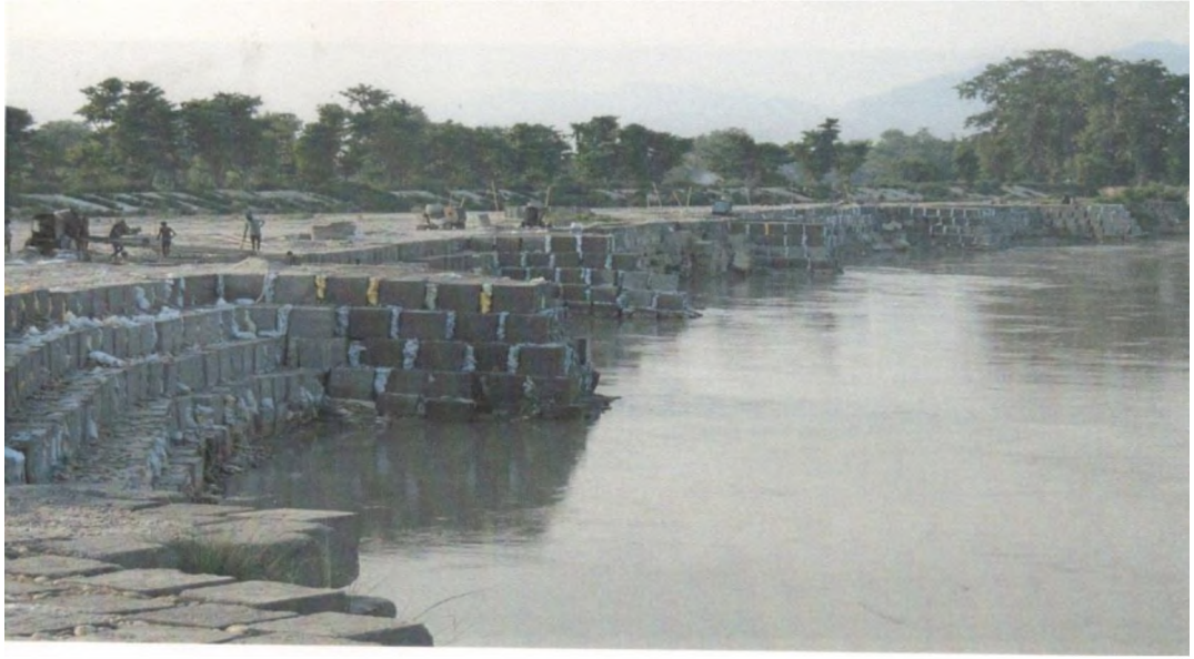
Protection Work in Gandak River, Nawalparasi, Nepal
