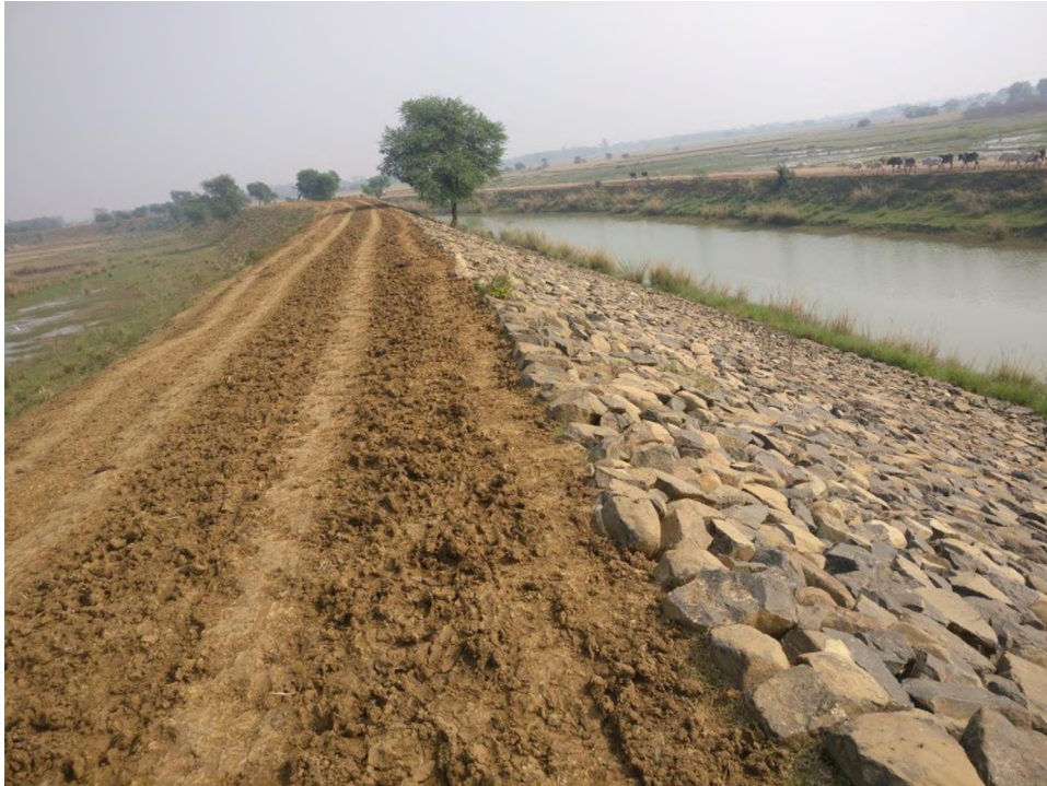
Anti Erosion work in Kandi Project, West Bengal
