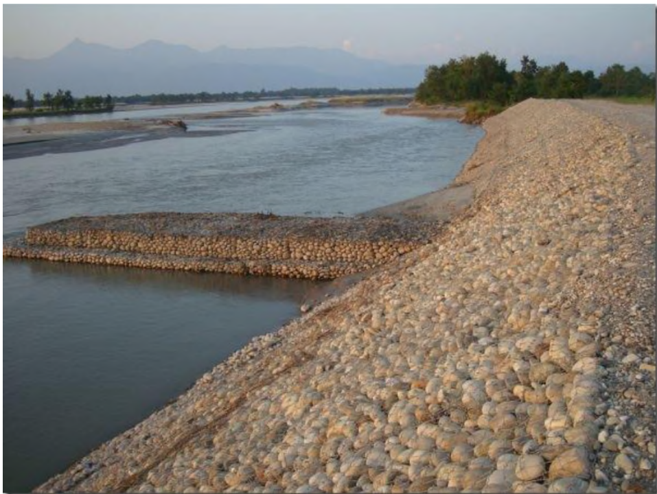
Anti Erosion works on Narayani Chittoni Embankment, Uttar Pradesh
