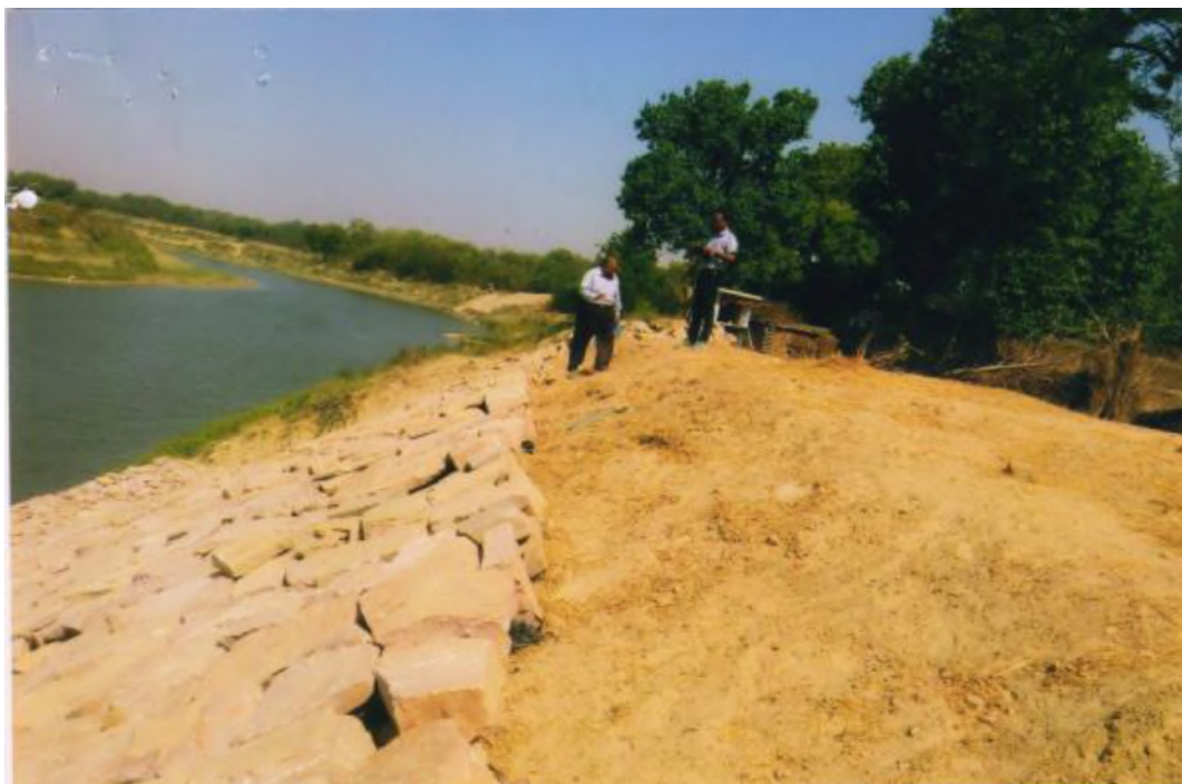
Bank Protection in Deoria, U.P.-24 Scheme
