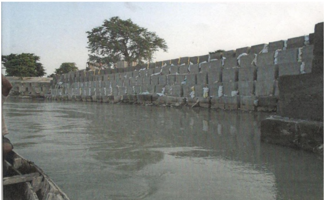
Protection Work in Gandak River, Nawalparasi, Nepal
