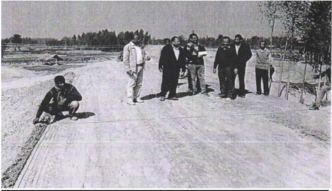
Elgin Bridge Embankment(UP-27)- Barabanki(U.P.)
