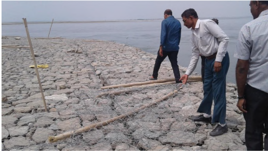
Measurement of a Launching Apron during Monitoring Visit
