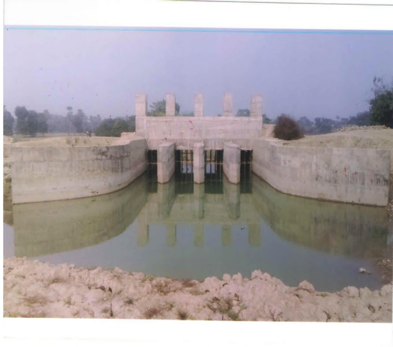
Anti Flood Sluice, Mohanpur UP
