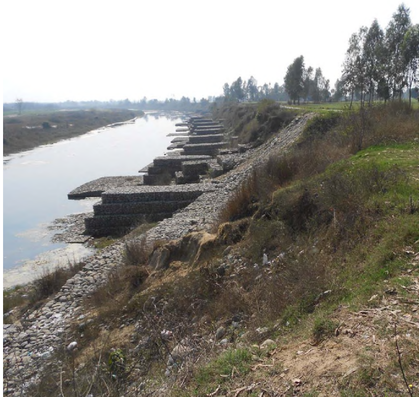
Anti-Erosion Works in Mohammadganj, Uttarakhand
