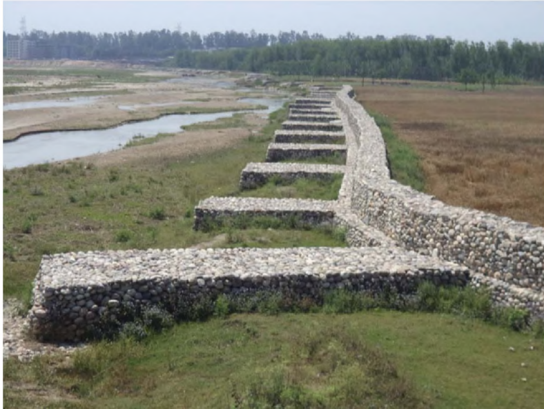
Bed bars constructed with gabions
