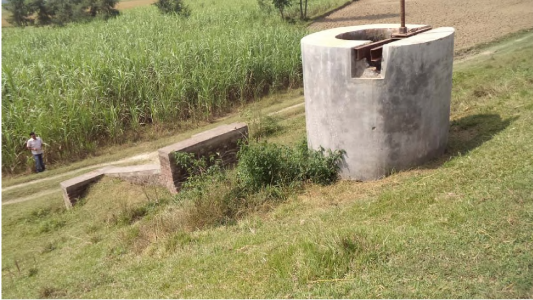
Anti-Flood Sluice constructed on Embankment
