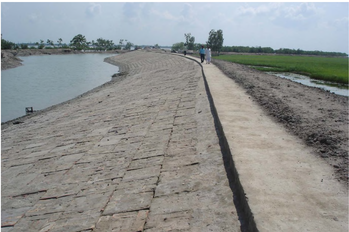
Anti-Erosion Works (Revetment) in West Bengal
