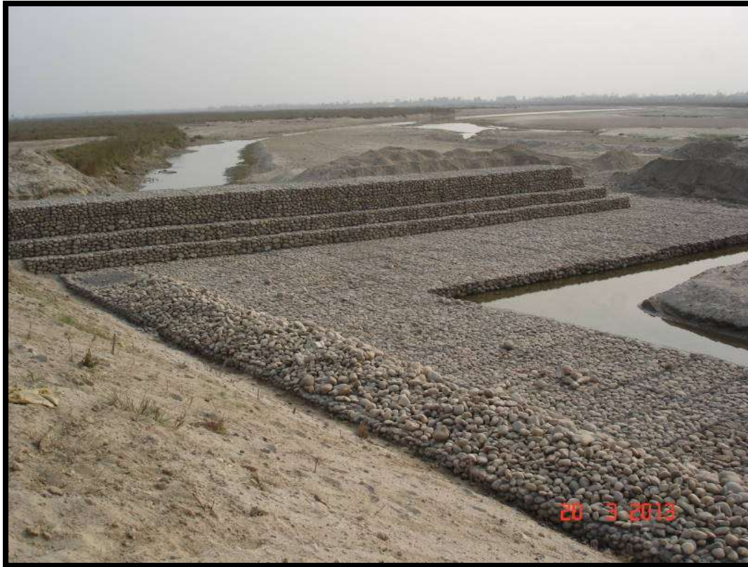
Anti-Erosion Works (boulder spurs) constructed on river Kamla in Nepal with funding from Government of India
