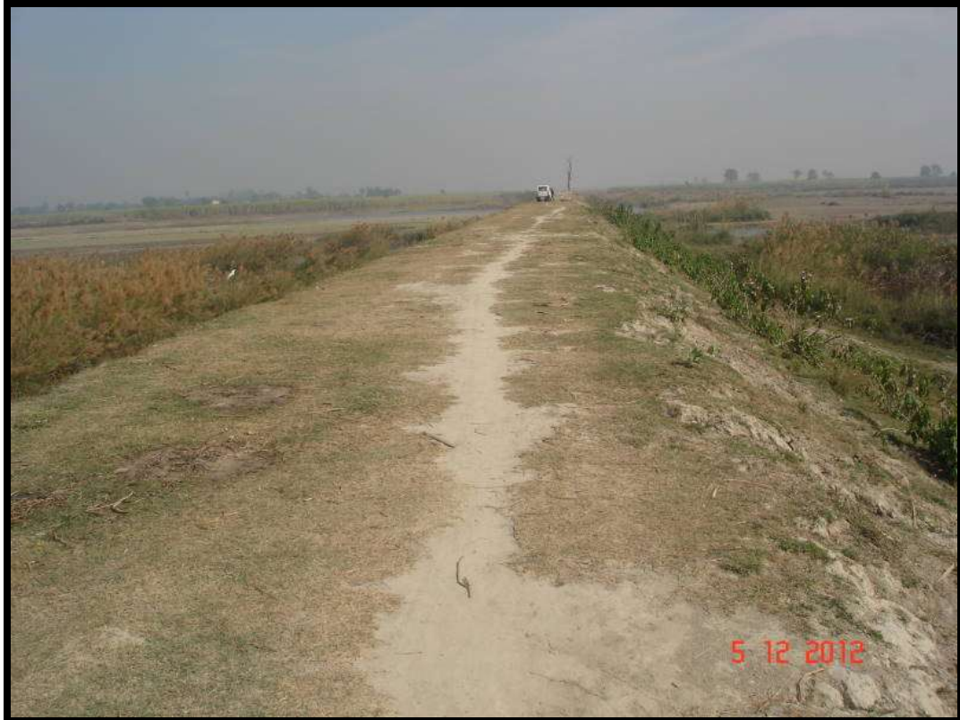
Construction of embankment on river Ganga in District Haridwar
